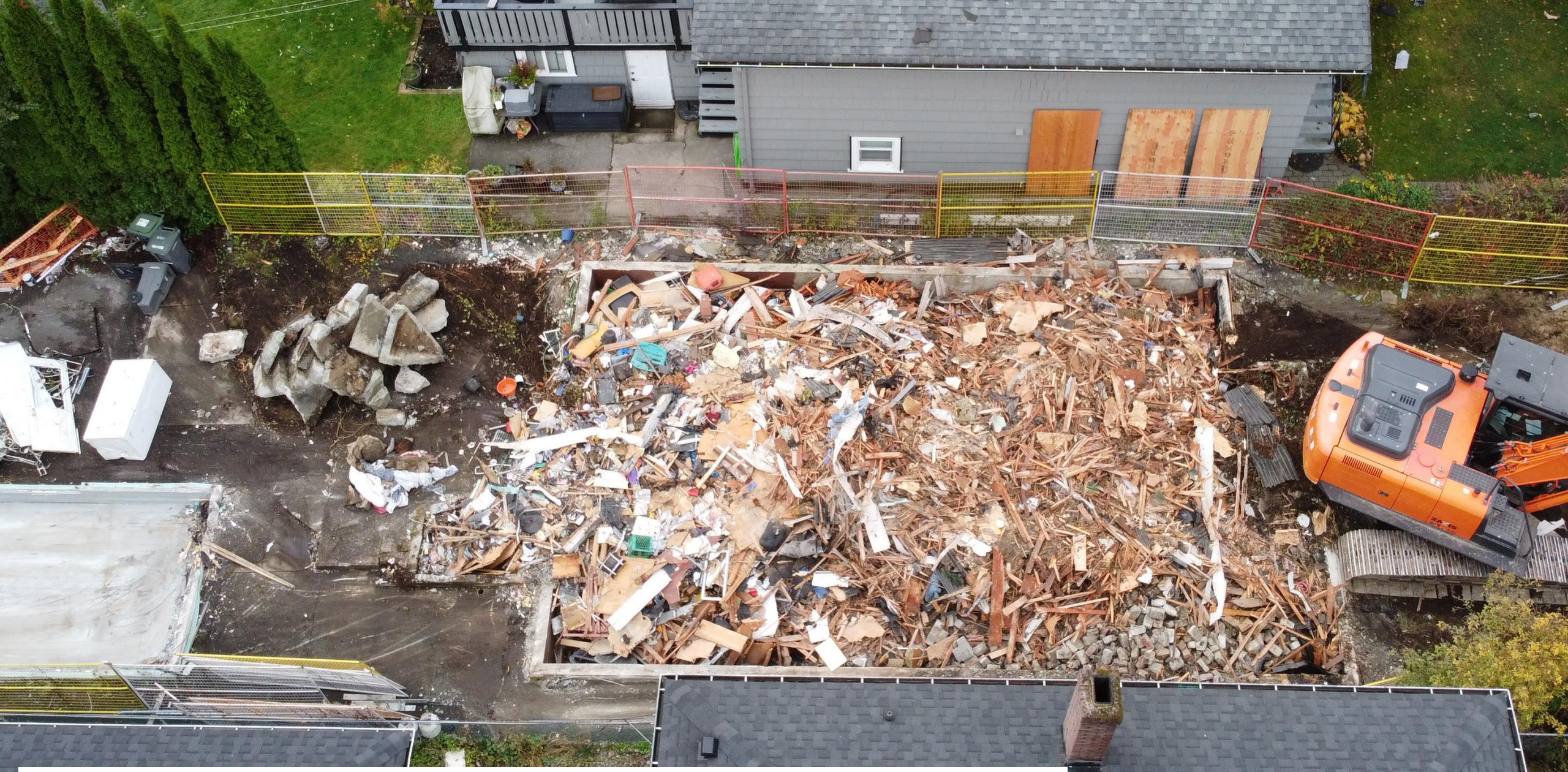
Urban woodwaste from residential demolition, Vancouver
